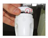
2) Rotate the limiter ring. Using the "T" notch as a reference (see figure), connect the ring in line with one of the 3 icons on the back of the handwheel:
