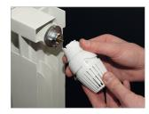
**3)** Unhook the thermostatic head with a light strength.
